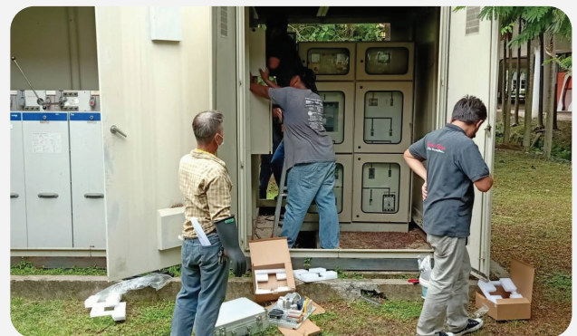
▲ Battery energy storage system installation
