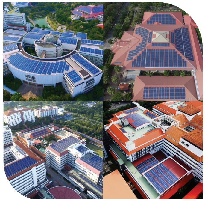
● Installation of Solar Rooftop
